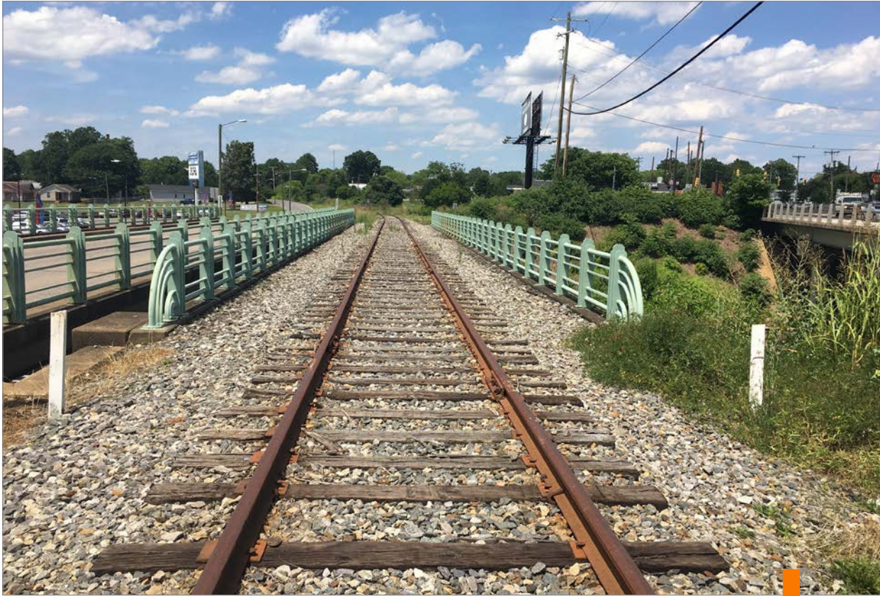
BRIDGE OVER US 74 (existing, south of Uptown Shelby)
