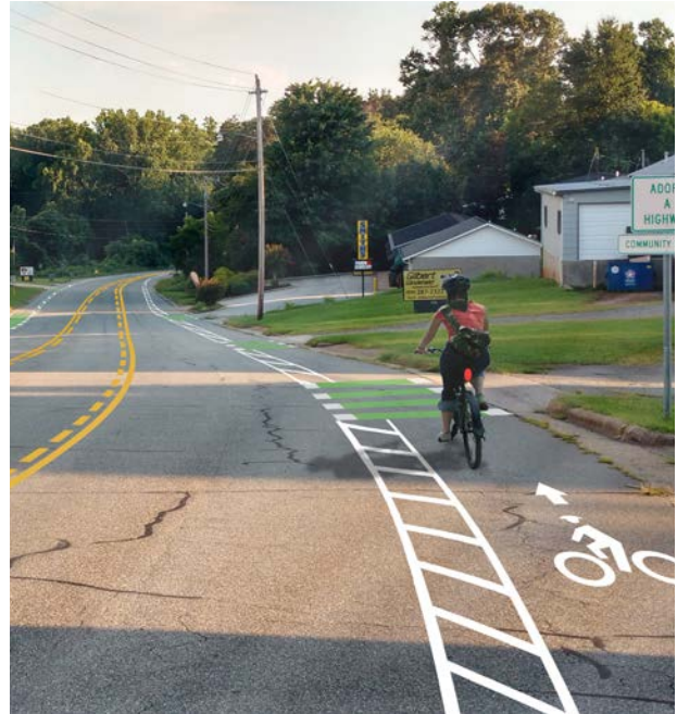
Example lane-reconfiguration recommendation: Oak Street in Spindale, NC (photo-rendering of "after" scenario).
